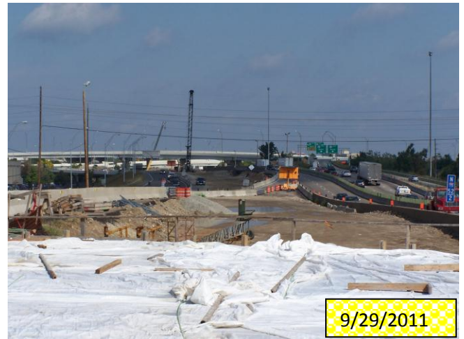
Looking north from the I-75 SB bridge over Stewart St.
