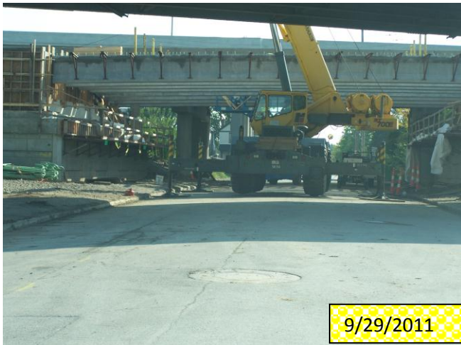
Looking east at the I-75 SB bridge over Albany St.
