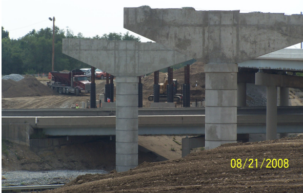
The new SR 4 flyover bridge piers
