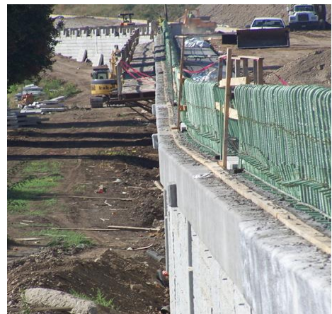
Looking at crews working on MSE walls.
