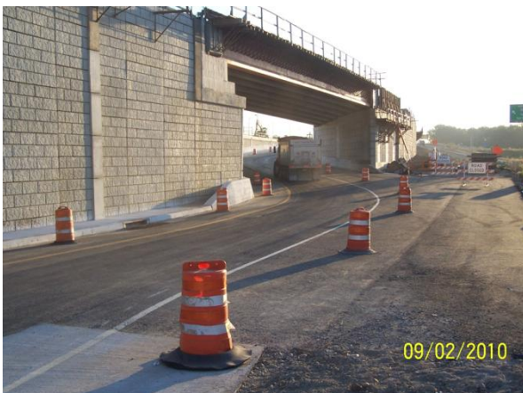
Looking at the new Main Street on ramp to I-75 northbound.
