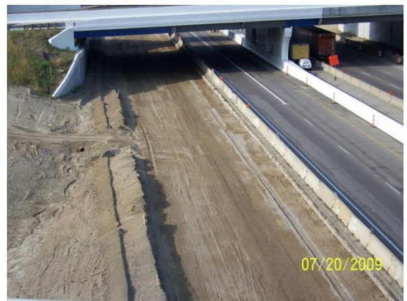
Looking south at I-75 NB just north of I-70.
