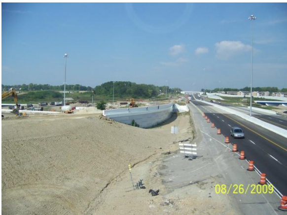
Looking west at the future ramp of I-70 EB to I-75 NB (top) and part of the closed old ramp (bottom).
