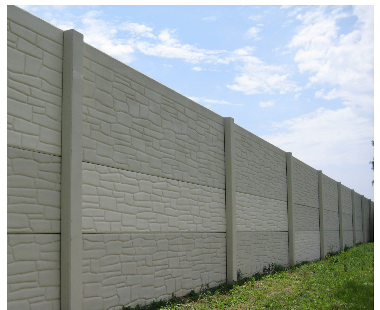
Noise Barrier Example
