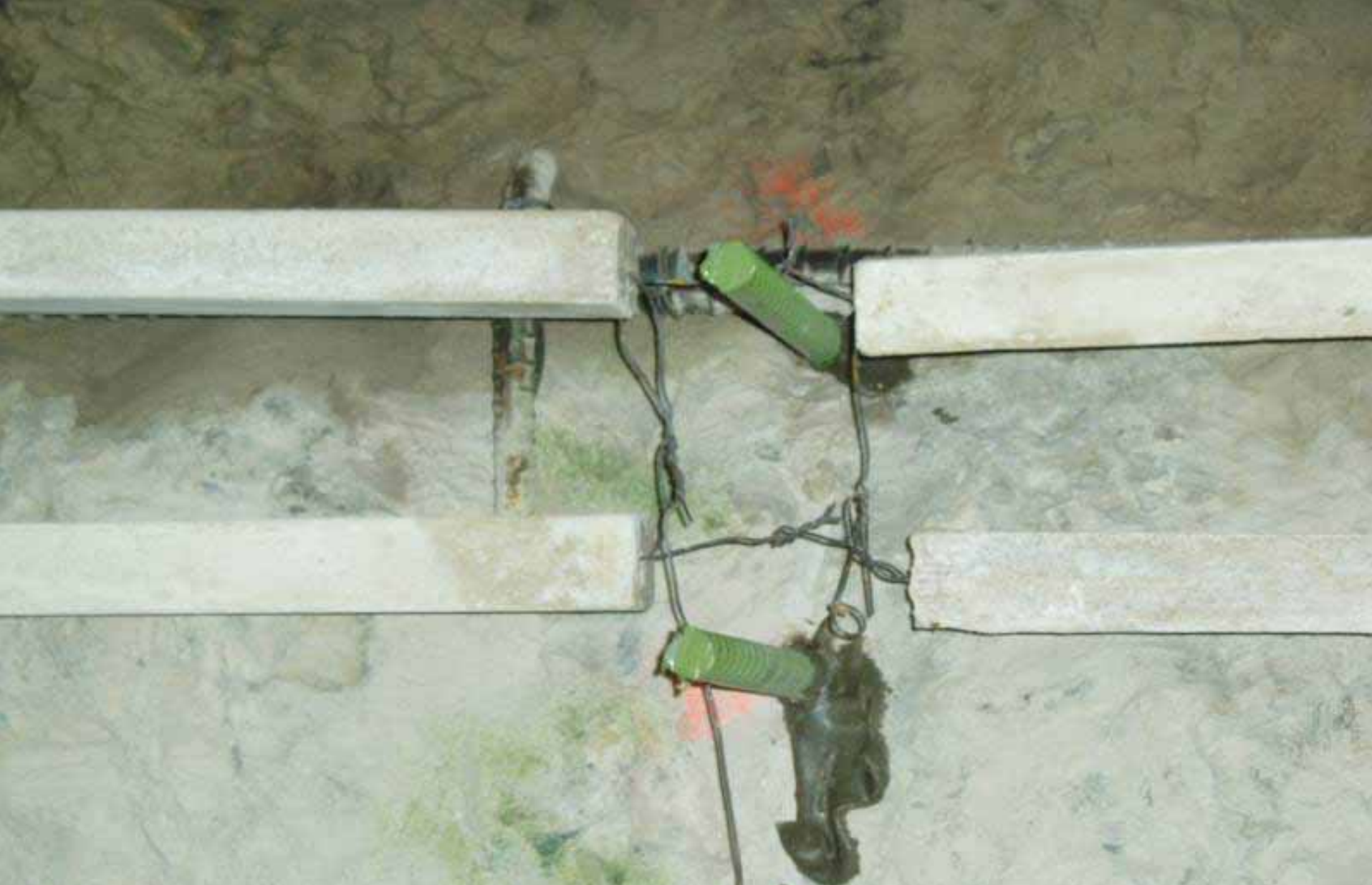
Connection of Anodes to Rebar
