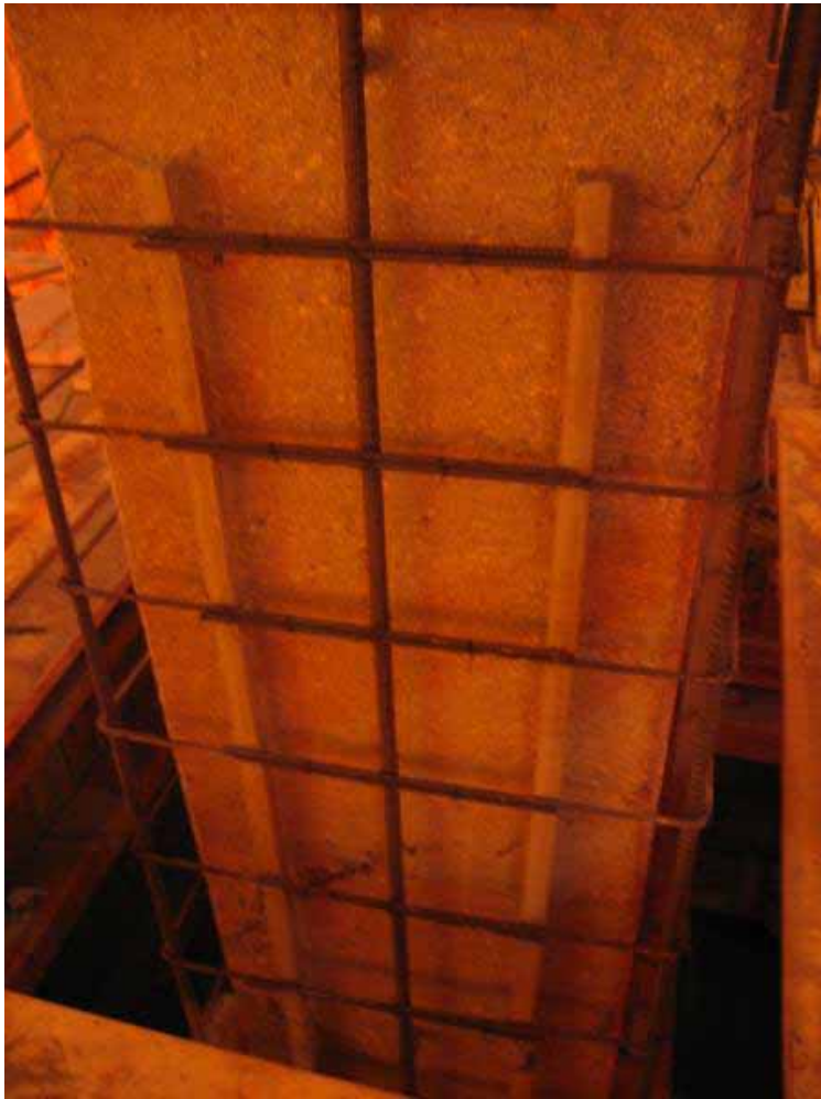
Bridge Column Repair with Reinforced Concrete Jacket
