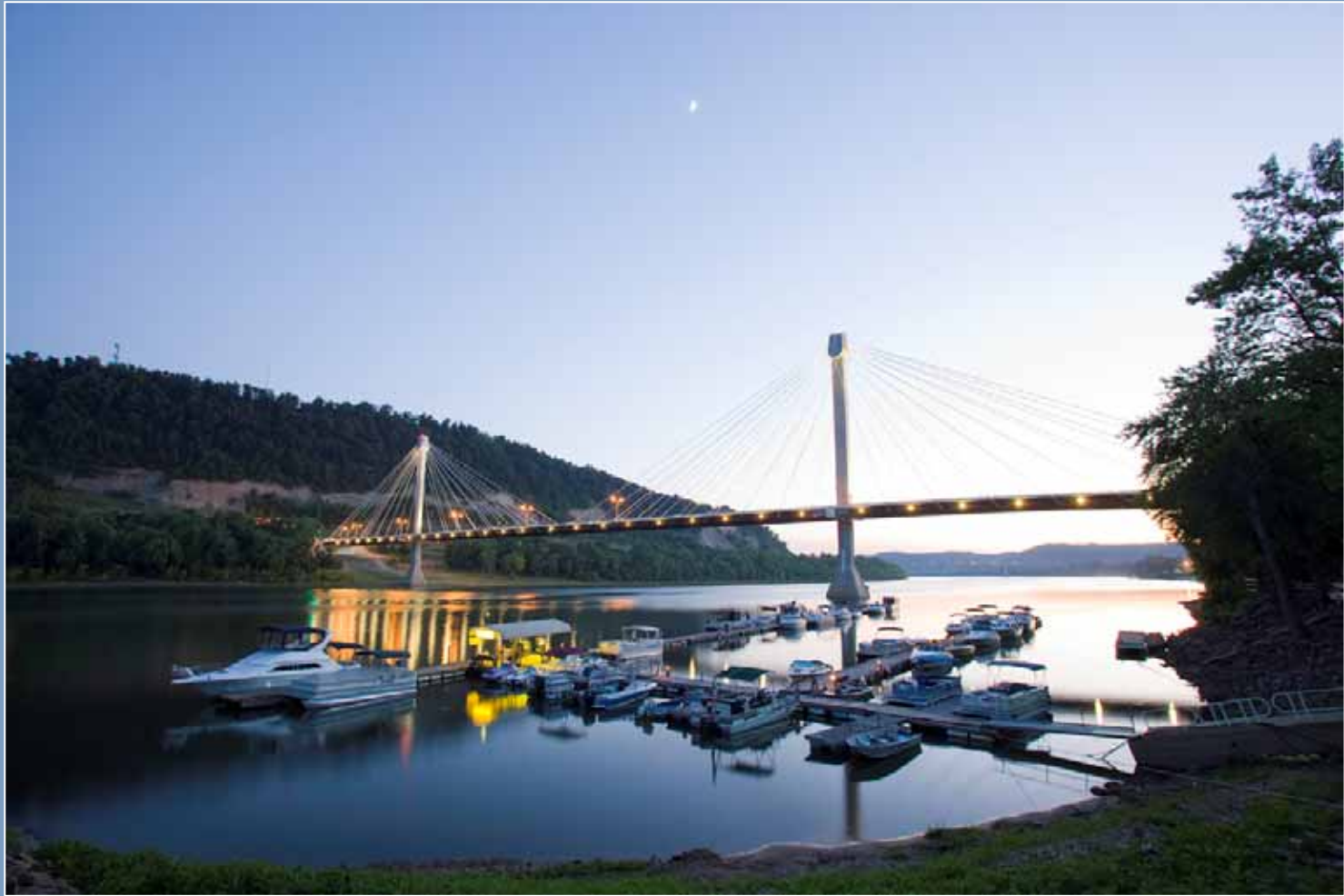
U. S. Grant Cable-Stayed Bridge
