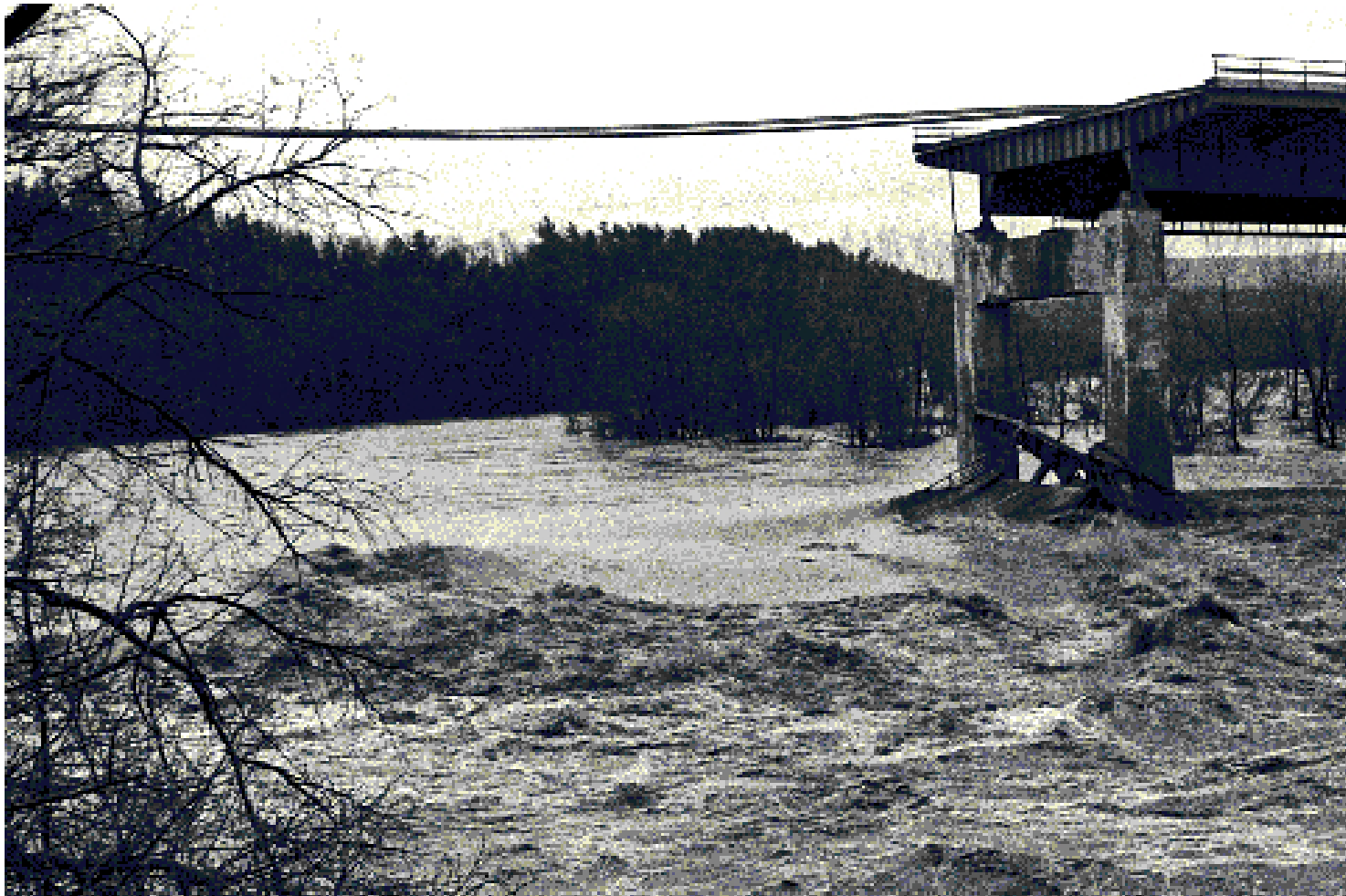
I-90 bridge collapse on Schoharie Creek, April 5, 1987. Courtesy of Sid Brown, Schenectady Gazette.
