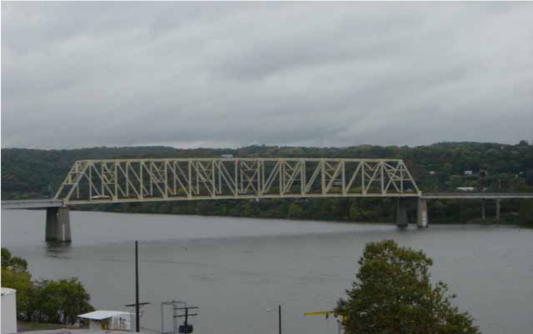
JENNINGS RANDOLPH BRIDGE
