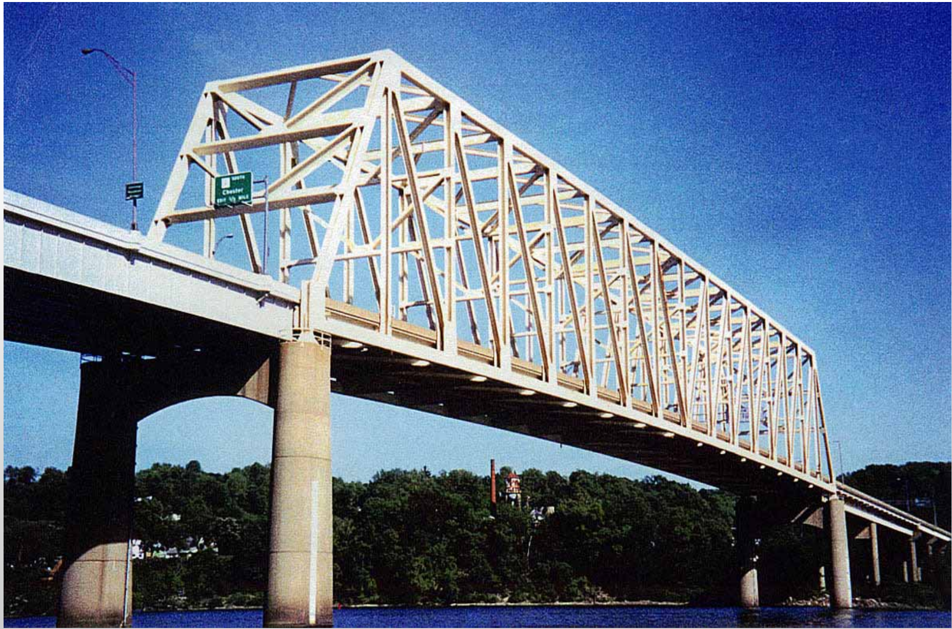
JENNINGS RANDOLPH BRIDGE
