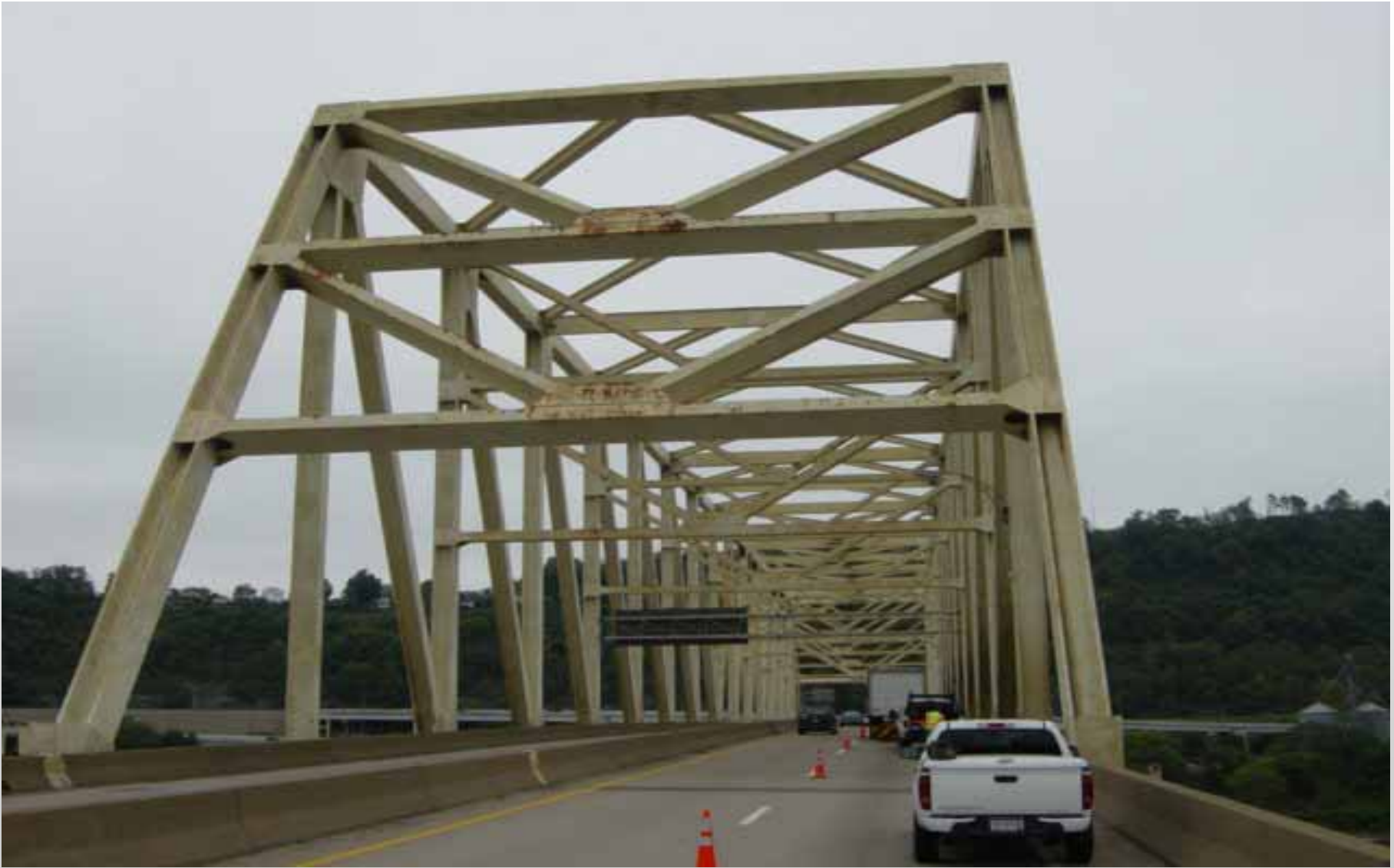
JENNINGS RANDOLPH BRIDGE
