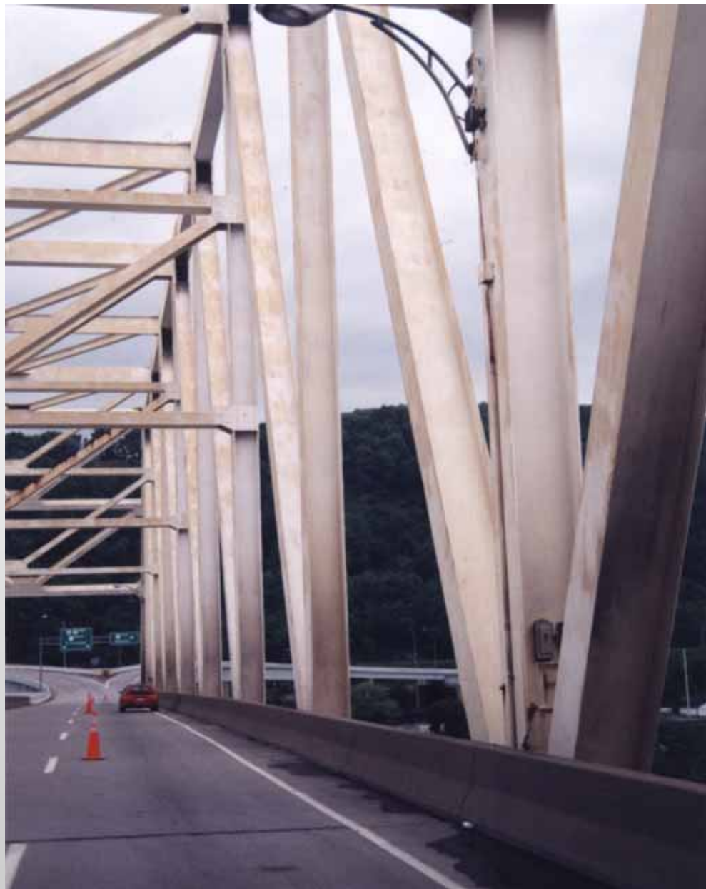
JENNINGS RANDOLPH BRIDGE (INSIDE)
