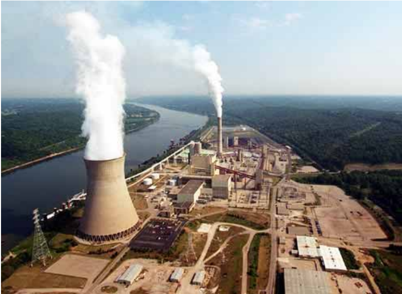
Zimmer power plant in Moscow, Ohio.
