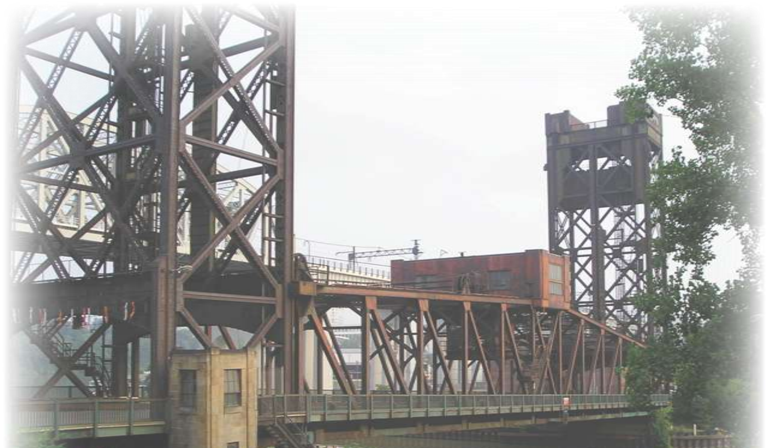
Columbus Road Lift Bridge Cleveland, Ohio
