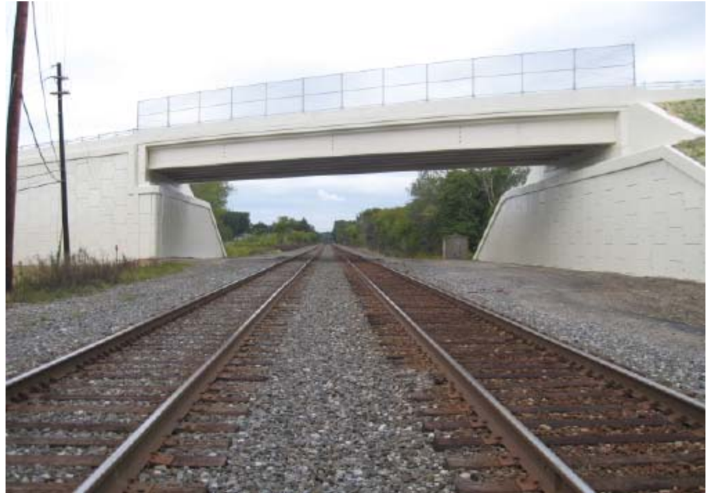
ODOT Grade Separation Program Geneva, OH – Austin Road
