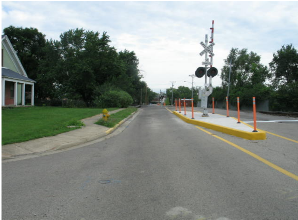
Union Street Signal Upgrade – Troy, OH
