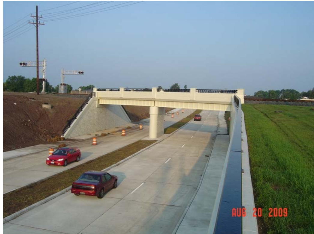
Snow Road Under Grade Separation
