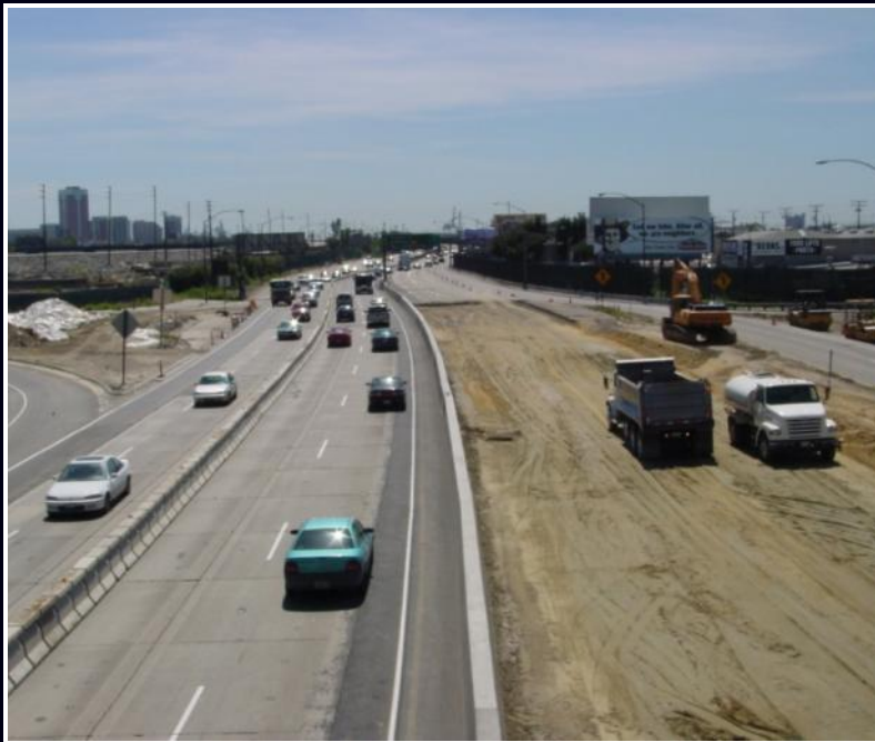
Partial Road Closure with Moveable Median
