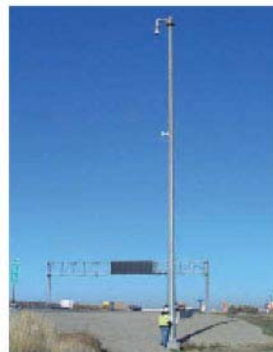
Cameras can be installed at any height to provide a greater field of view as height is not limited to the reach of large bucket trucks
