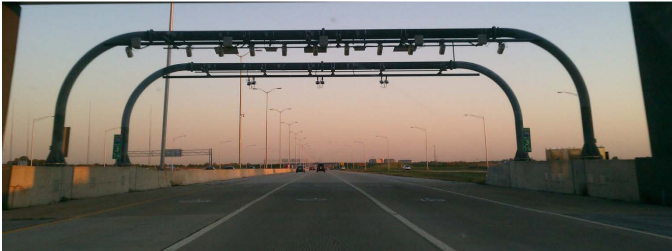
View from Vehicle Approaching a 3 Lane ORT Zone
