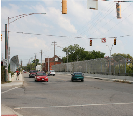
View of the existing bridge looking north.
