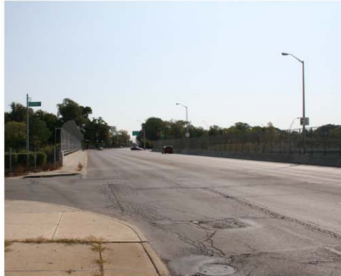
View of the existing bridge looking east.
