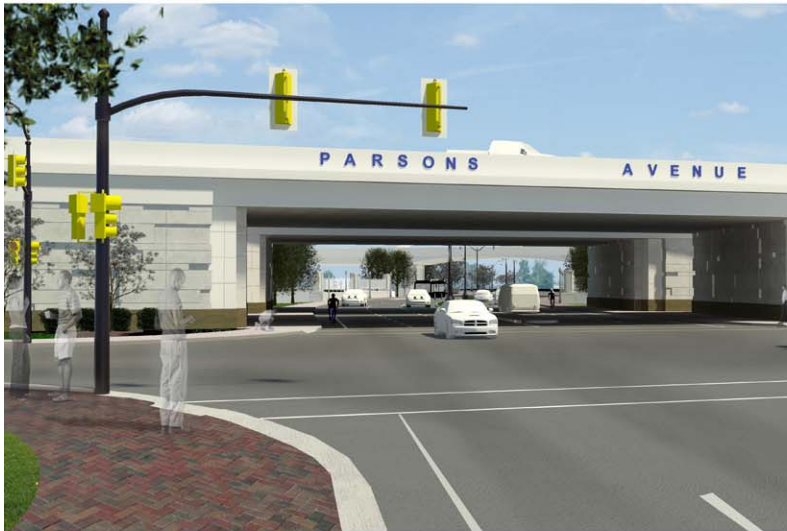
View looking north along Parsons Avenue at the intersection of Mooberry Street. I-70 is crossing on the bridges above Parsons.
