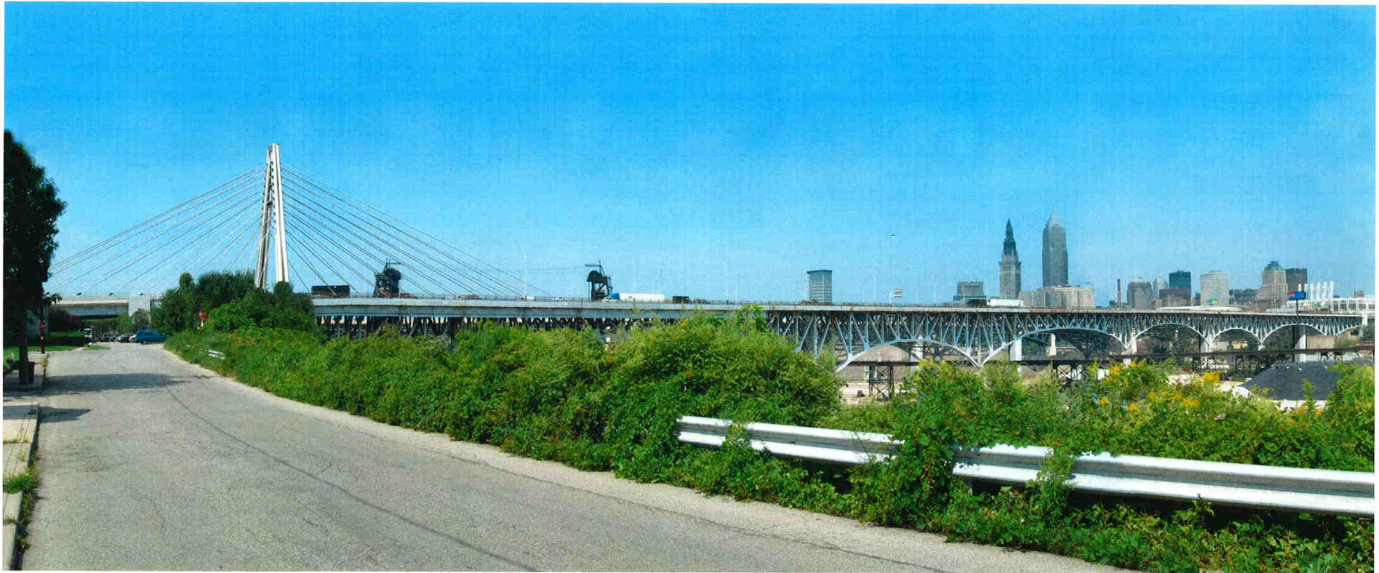
Rendering of New Westbound Bridge Existing Bridge in Service for Eastbound Traffic
