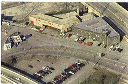
Aerial View of Rescue Station & Fire Museum
