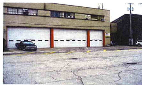
View Facing Rescue Station from Commercial Road
