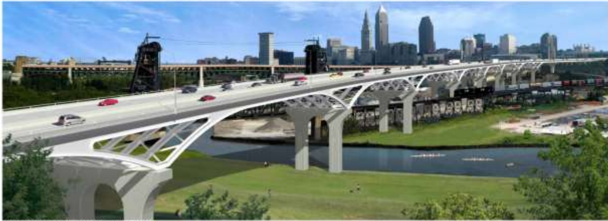
I-90 VIADUCT BRIDGE - VIEW (1) LOOKING NORTH (DAY)
