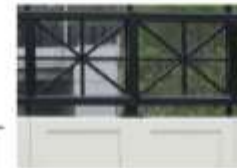
DECORATIVE RAILING - PHOTO FROM ABBEY AVENUE OVER GCRTA
