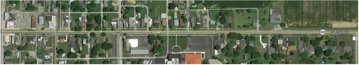
Existing Main Street in Arlington Phase 2, prior to construction.
