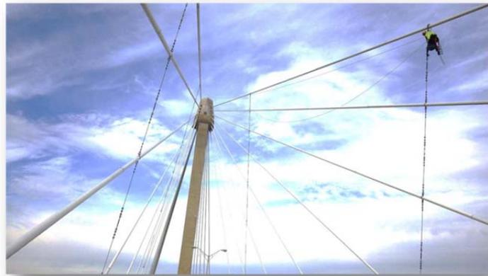
Figure 45 - Inspector Rappelling the Cable Stay
