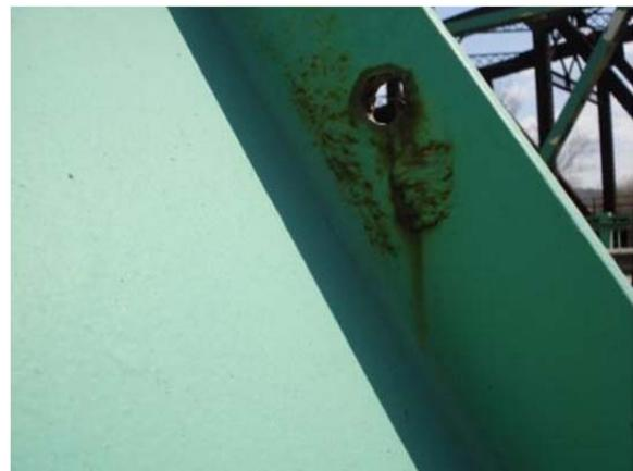
Figure 38 - Plug Weld
