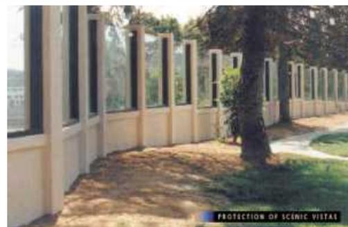
The visual character of noise barriers in relationship to their environmental setting should be carefully considered. In general, it is desirable to locate a noise barrier approximately four times its height from residences and to provide landscaping near the barrier to avoid visual dominance. Noise barriers should reflect the character of their surroundings as much as possible. It is always desirable to preserve aesthetic views and scenic vistas, to the extent possible.
