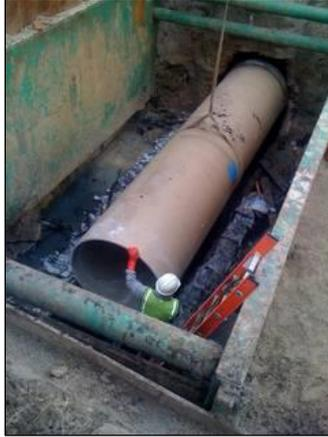
Figure 2-15. Segmental sliplining method (Source: Hobas Pipe USA).
