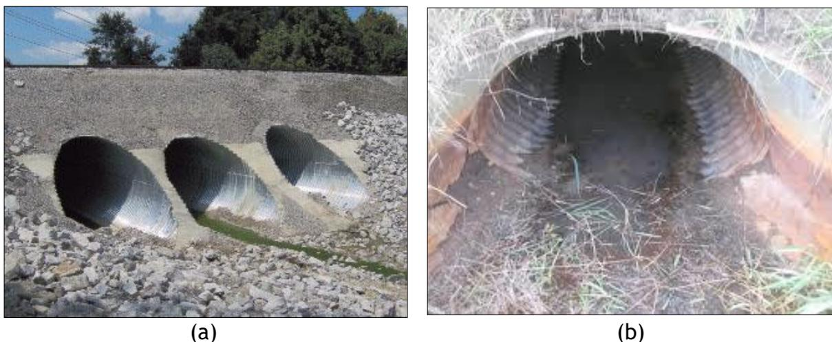
Figure 2-2. Corrugated metal pipe culverts (CMPs): (a) multi-cell CMPs (Source: Contech) and (b) invert deteriorated CMP (Source: Metal Culverts, Inc.).
