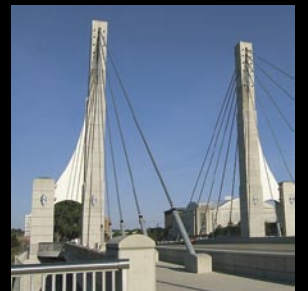
Example from Columbus, OH (Lane Avenue Bridge)
